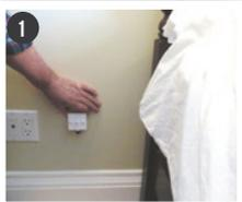
At wall socket location in bedroom, remove white screw caps from wall socket, then remove face plate (retain screws and caps) place 4 - #6x2.1/2 screws provided through holes in wall socket, locate on wall in location required and insert screws 2 or 3 turns into wall to mark locations for anchors. Remove screws and insert anchors provided into wall.
