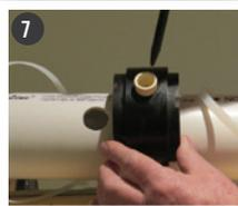
Drill 1" dia. Hole through wall of sanitary pipe, we recommend a 1/8" dia. Pilot hole first. Place plastic ties provided in a loop around sanitary pipe (do not tighten ties).
