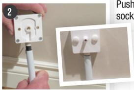
Push end of Pex U-drain line firmly onto wall socket stub and affix to wall.
