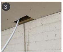
Run the Pex to sanitary/saddle location maintaining min. 1/8" per foot slope (more severe slopes or vertical drops are acceptable). Avoid creating pockets where liquids can collect in pipe. We strongly recommend using a wall anchor on pex pipe as close to wall socket as is acceptable.
