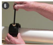
Hold saddle on upper half of horizontal sanitary pipe, push pencil through saddle stub and mark location of 1" dia. Hole to be drilled in sanitary pipe. For vertical sanitary pipe, saddle can be located on any part of circumference.
