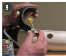
Apply all-purpose cement to Contact Side of Saddle and re-fit on sanitary pipe, immediately tighten one tie at each side of stub and allow cement to dry 30 min.
