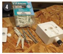
Attach wall socket to wall using 4 - #6 x 2.1/2" screws provided. Make sure valve is intact in wall socket.
